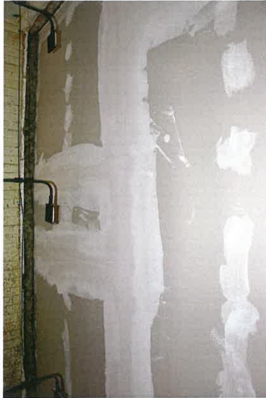
Photo No. 26924d-03: Exposed side of the specimen before the test
