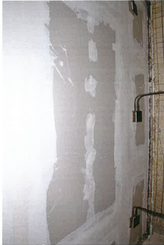
Photo No. 26924d-01: Exposed side of the specimen before the test
