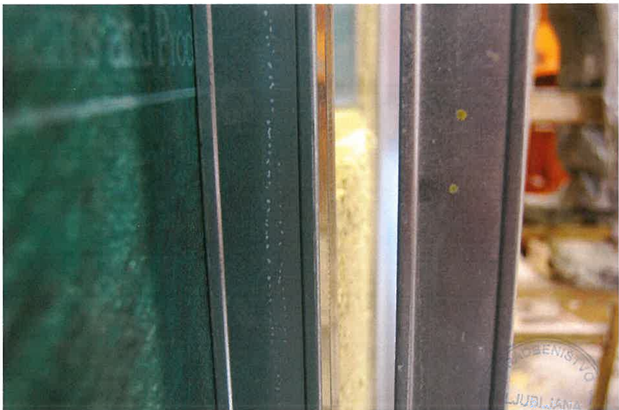
Photo No. 26932d-06: Gap between frameworks
